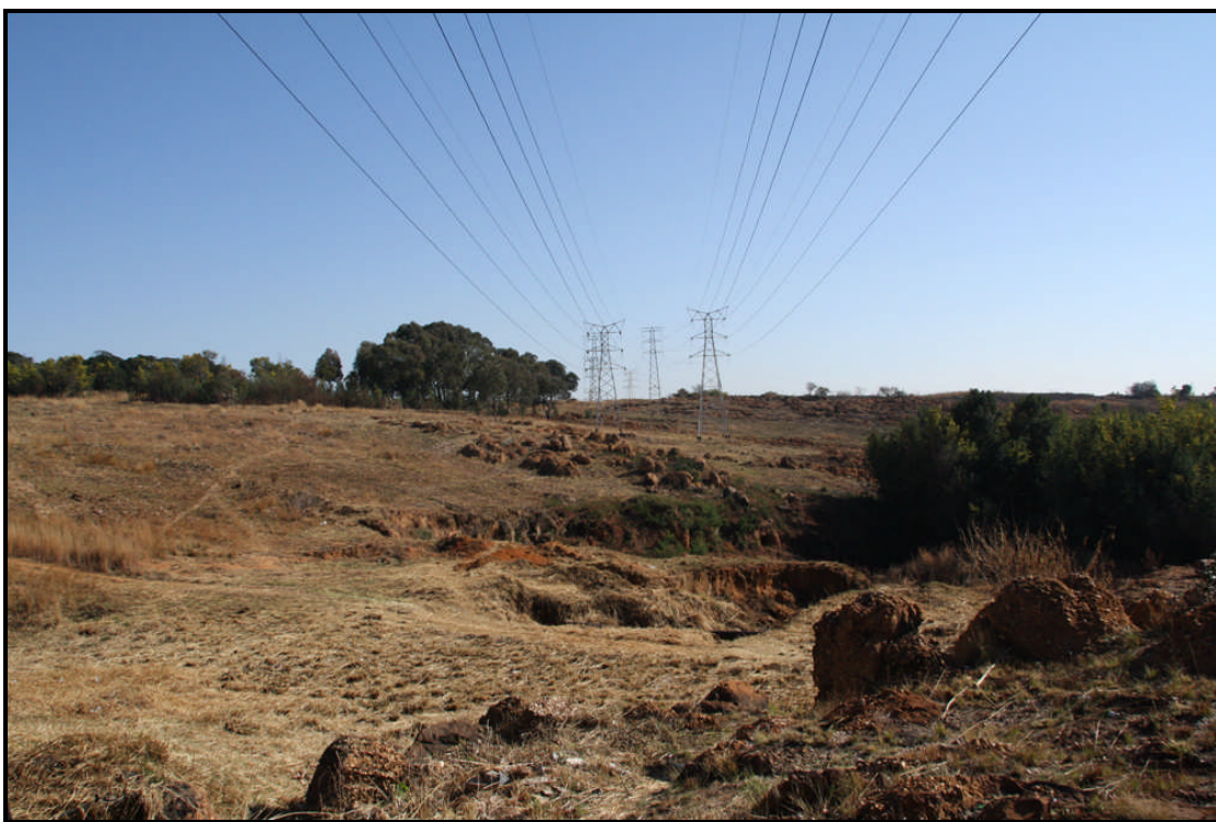
Fig. 11. The stream bed below the Eskom power line.
