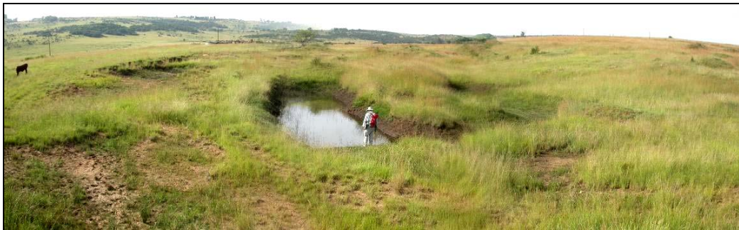
Figure 8: View south at southwest corner of the site, showing a pond formed in an excavated pit and associated seepage/drainage to the left foreground.
